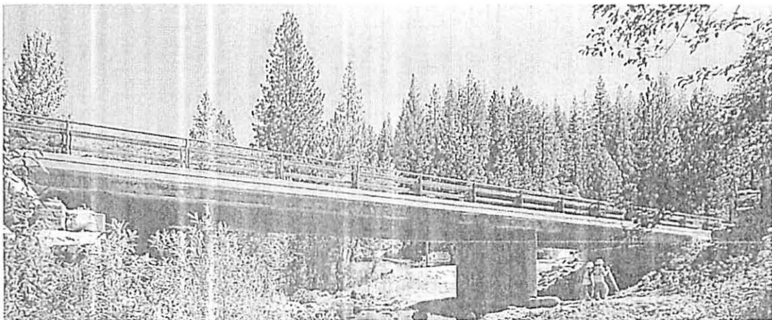
New Hayfork Creek Bridge on Wildwood Road—June 2016
