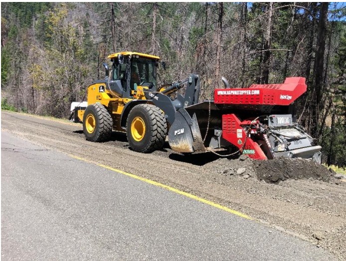
July 2023; Ruth-Zenia Road repairs by County crews (grinding & removing damaged materials)
