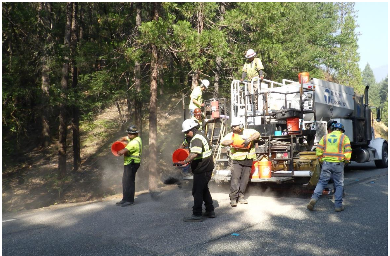
High Friction Surface Treatment, workers augmenting the surface with additional chips
