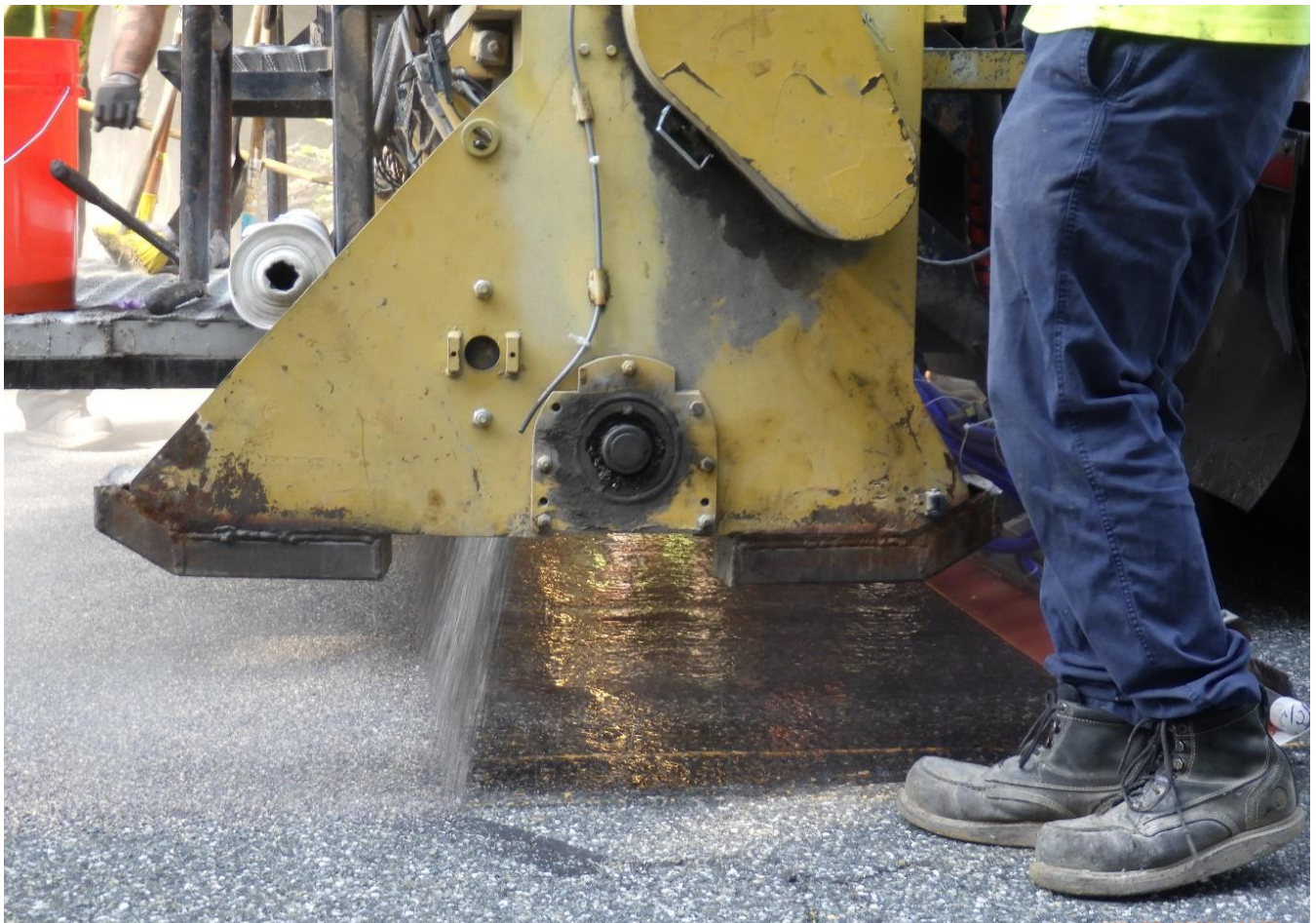
High Friction Surface Treatment with bonding agent(glue) and chip application
