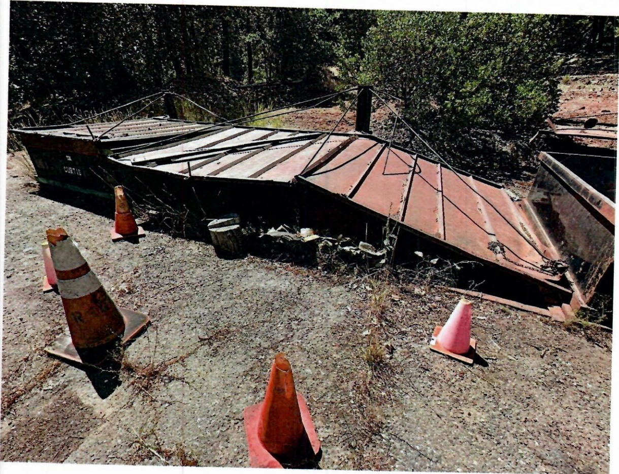
Figure 2. Hyampom Transfer Site. Abandoned inground bin pockets
