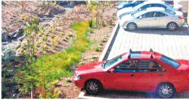
A daylight stream, a rain garden, porous pavement, and native plants all work together to protect water resources on and off site.
