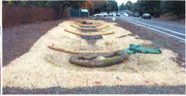
Even a single practice like this rain garden will need additional BMPs implemented (erosion control) to be really effective long-term.
