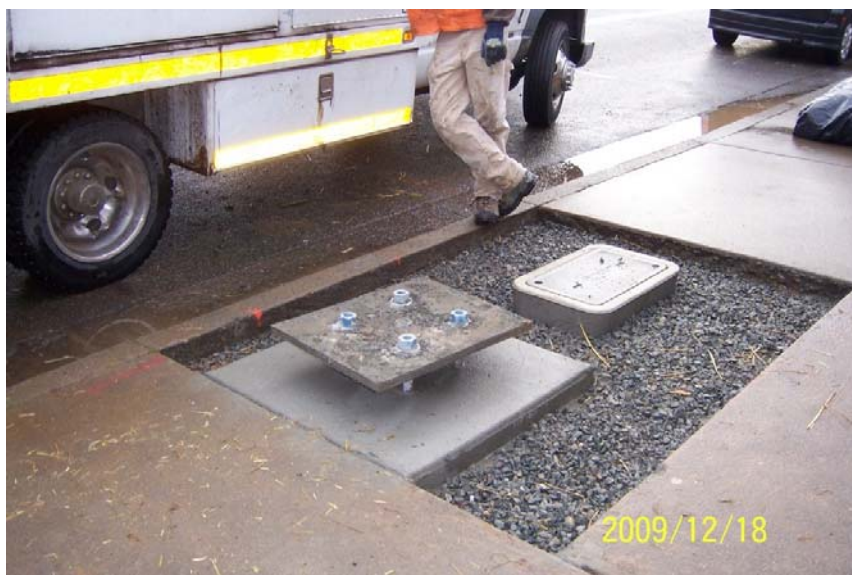
Ready to Place Sidewalk Concrete Around Pole Foundations
