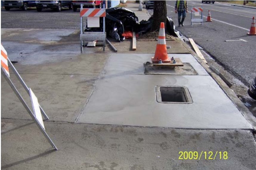
Foundation and Sidewalk Nearly Complete
