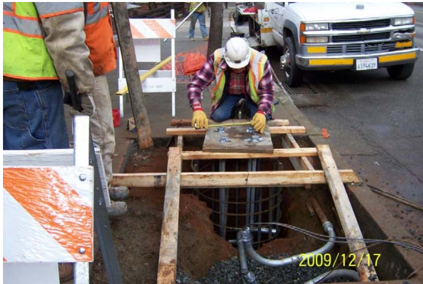
Forming Foundations and Setting Anchor Bolts for Pole
