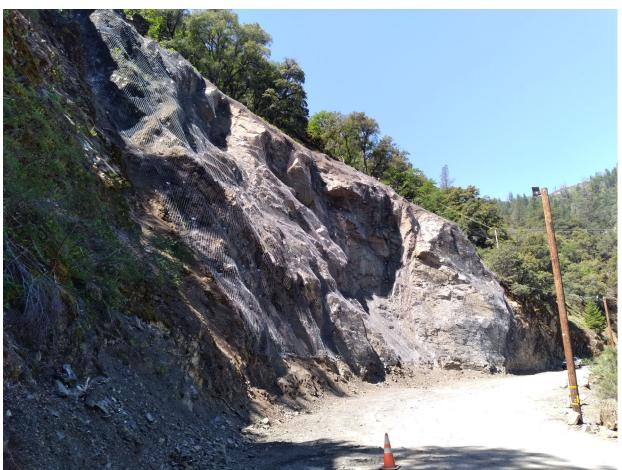
Canyon Creek Road, final rock slope repairs using grouted anchors and steel net to stabilize the slope
