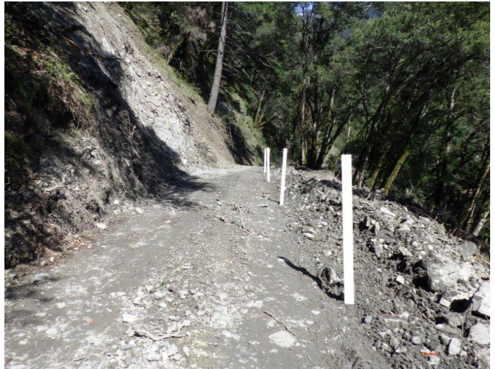
Fisher Road (one lane rd.) storm damage above, repairs and final opened road below with edge markers
