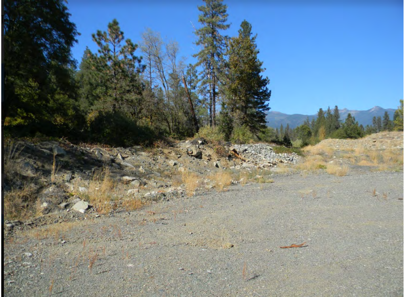
FIGURE 6. LEVEE SEPARATING ADJACENT RIPARIAN HABITAT AT 311 INDUSTRIAL PARK WAY, WEAVERVILLE, CA.
